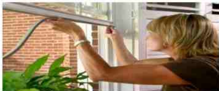
Fig. 5 Lady implementing Weatherstripping
